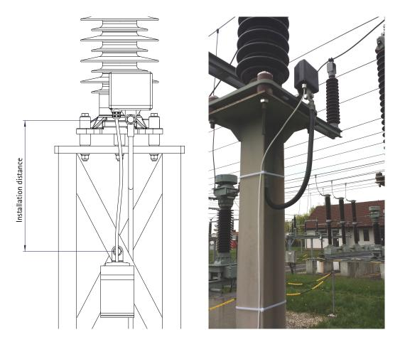
The data cable is weather- and UV-resistant and made for outdoor installation. We do not recommend to lead the cable through pipes or canals to prevent cable damages and influences to the data transmission.
