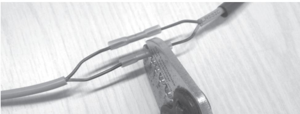
Pull the heat-shrink hose (1) over joint so that it covers completely. Heat the heat-shrink hose (1) with a blow-torch or heat gun.
